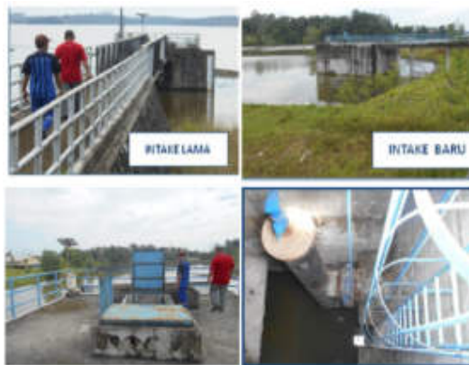
Figure 7 Dam Intake Conditions
