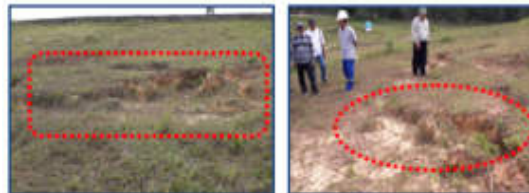
Figure 5 Downstream Slope Conditions of the Dam
