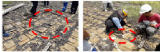
Figure 4 Condition of the Upstream Slope of the Dam
