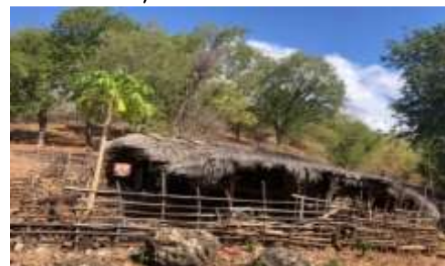
Figure 8. Condition of the garden house of one of the residents of RT 10 We'ain Hamlet, Kenebibi Village
