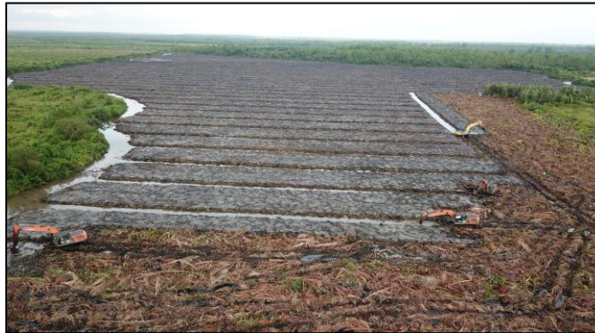
Picture. 2 Cambering Pattern Land Clearing Process
