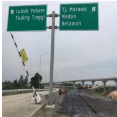
Figure 1. Lubuk Pakam – Sei Rempah Toll Road
