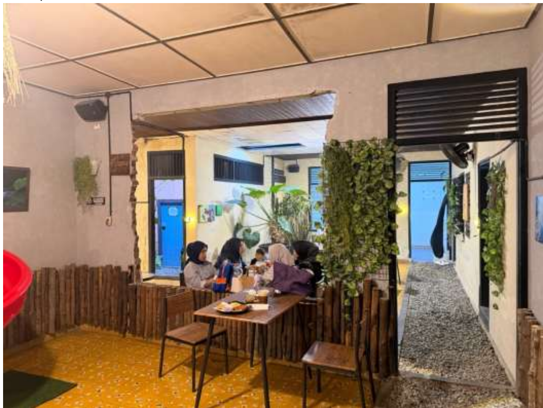
Fig.6. The interior configuration utilizes large openings to establish continuous spatial relationships between rooms. Partial removal of partition walls enhances visual permeability and reinforces the perception of openness within the space.
