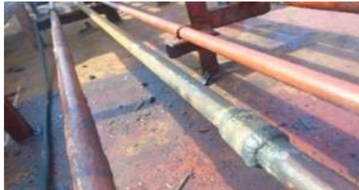
Figure 8. Reinstallation of Hydraulic Pipes
