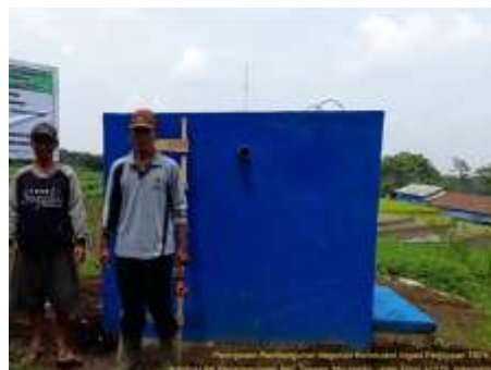
Image 4 : water reservoir construction completed
